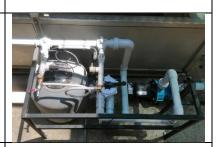
Stage #3 – Automatic Water Treatment Chemical Dosing System Supply and fit a ScaleAway ACDS to chemically treat the cooling water in cooling towers simultaneously.
